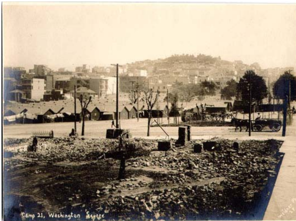
Figure 15. Earthquake refugee camp (Camp 21), Washington Square, 1906.
