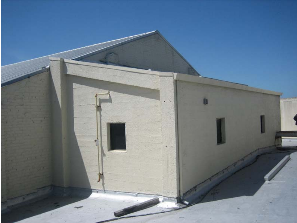
Figure 29. View of Projector Room from roof, April 2007. Source: Page & Turnbull, Inc.
