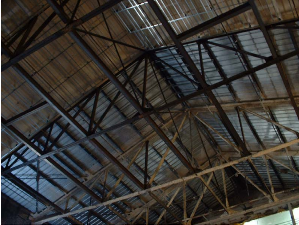
Figure 33. Interior, detail of trusses, April 2007. Source: Page & Turnbull, Inc.
