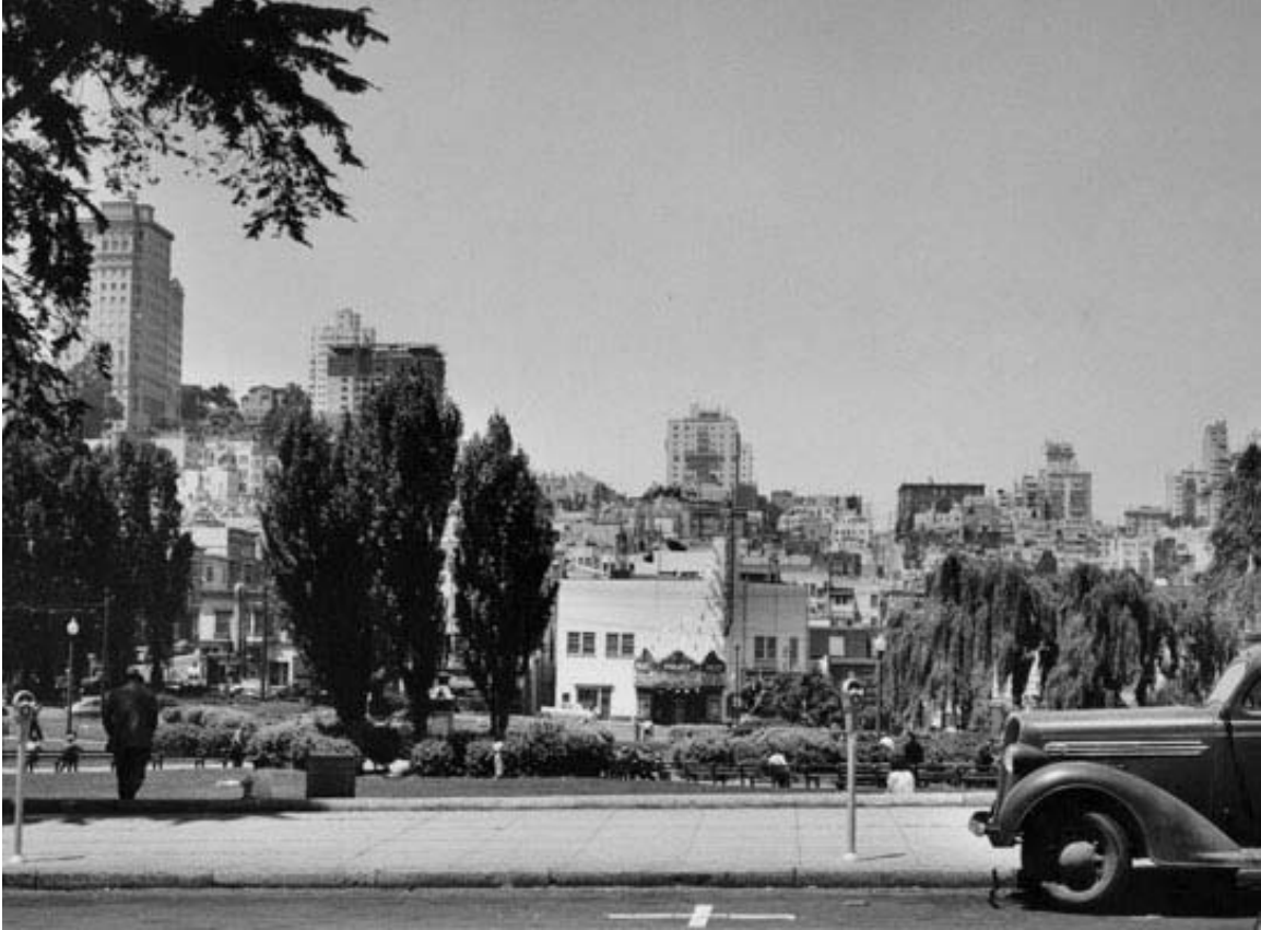
Figure 16. View of Russian Hill from Washington Square, n.d. Note Pagoda Theatre in the near background. Source: San Francisco Public Library Historical Photograph Collection
