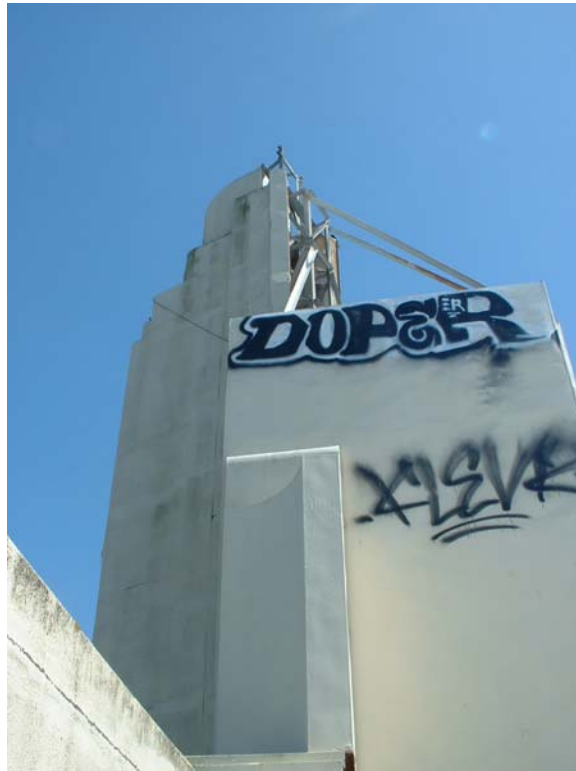
Figure 26. View of blade sign from roof, April 2007. Source: Page & Turnbull, Inc.
