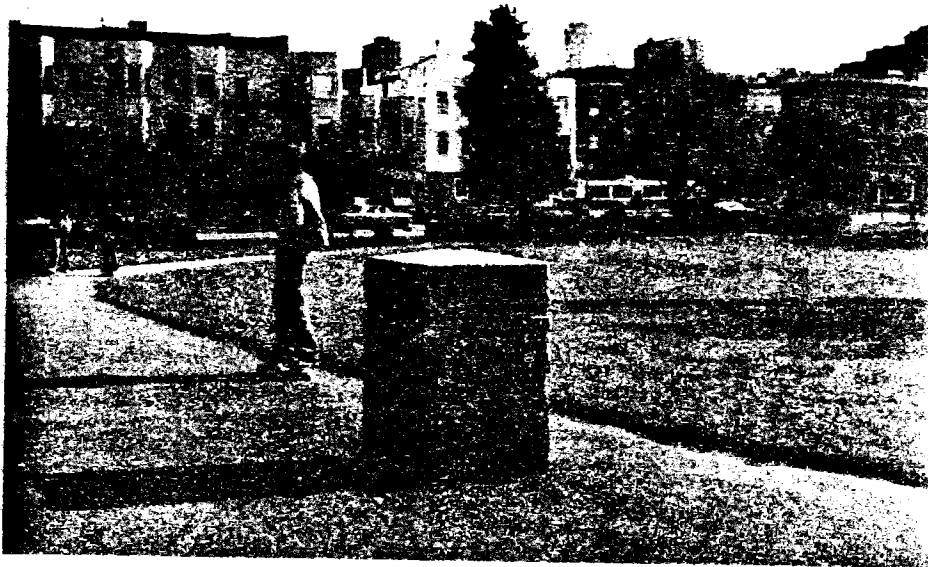
18b. Survey marker, Washington Square. Placed 1869; latitude & longitude carved 1937. Granite. It reads: "U.S. Coast & Geodetic Survey, Astronomical & Telegraphic Longitude Station Washington Square, 1869-1880; Latitude: 37.47'59" N, Longitude 122.24'37" W."
