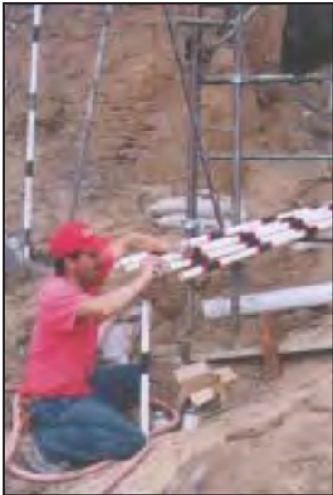
20,000 LF - Dana Point, CA project
