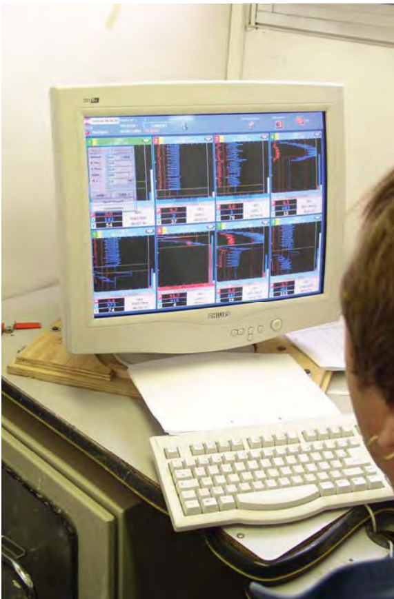
Figure 6.2.2-A: Computerized Grouting Display
