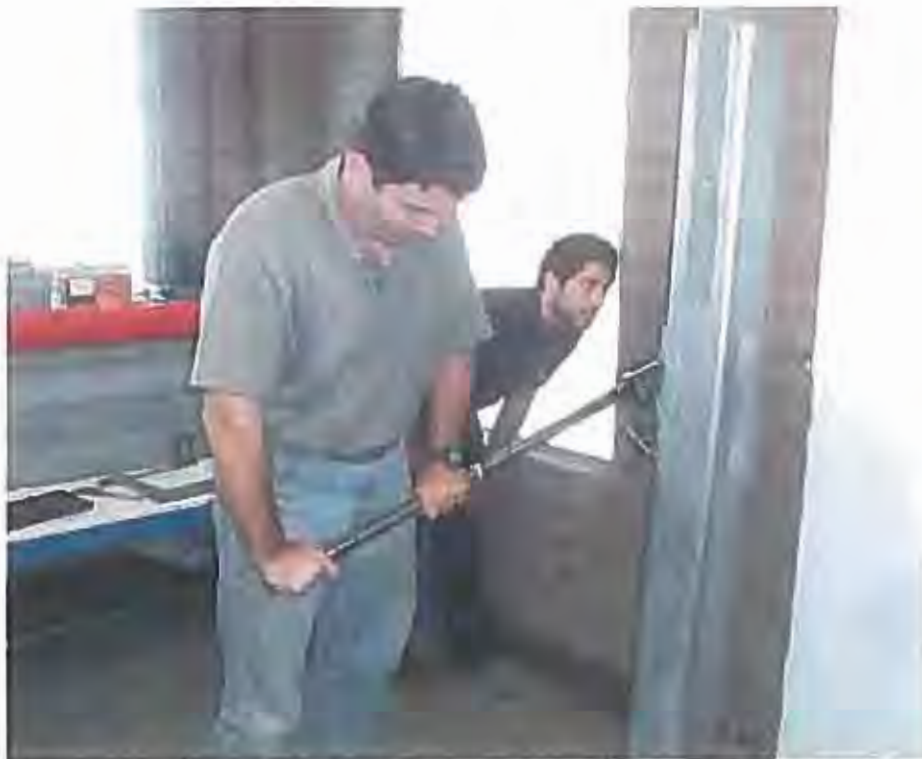
Figure 3. Bolt tensioning using wrench, tension read by technician
