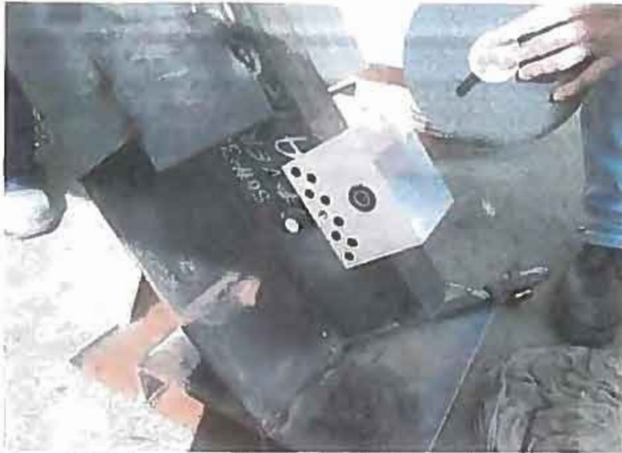
Figure 1. Mock up assembly with installed bolt and machining fixture
