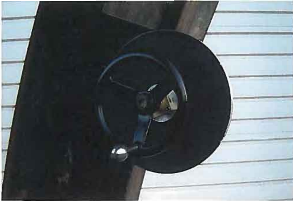
Bolt location "B"
