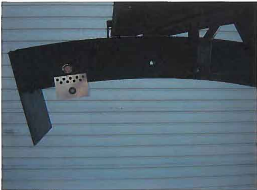
Bolt location "A"
