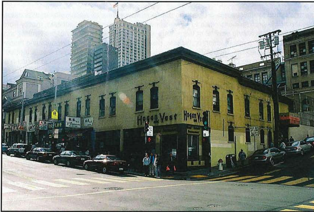
Figure 5.6. Existing building at 933-935 Stockton Street.
