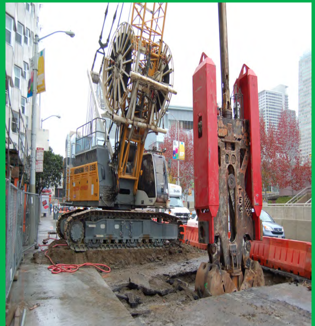
Excavation for the North Headwall at Yerba Buena /Moscone Station.
