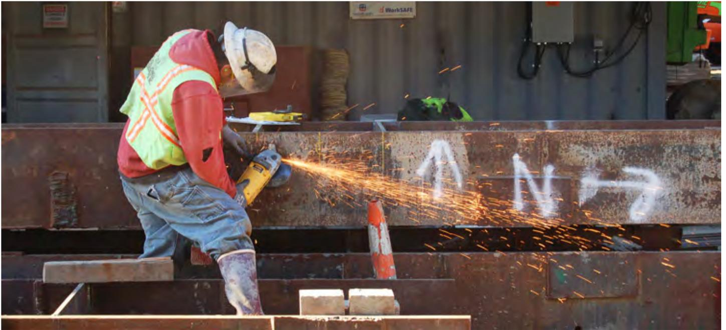
*A worker prepares the surface of a steel I-beam which will be used to brace the walls of the 4th Street launch box.*
