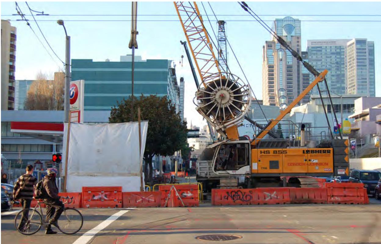
Crews use a crane and clamshell digger to excavate the future Yerba Buena/Moscone station headwalls, ahead of actual station construction which will take place under Contract 1300. The station entrance will be located on the site of the 76 gas station pictured here, photo left.
