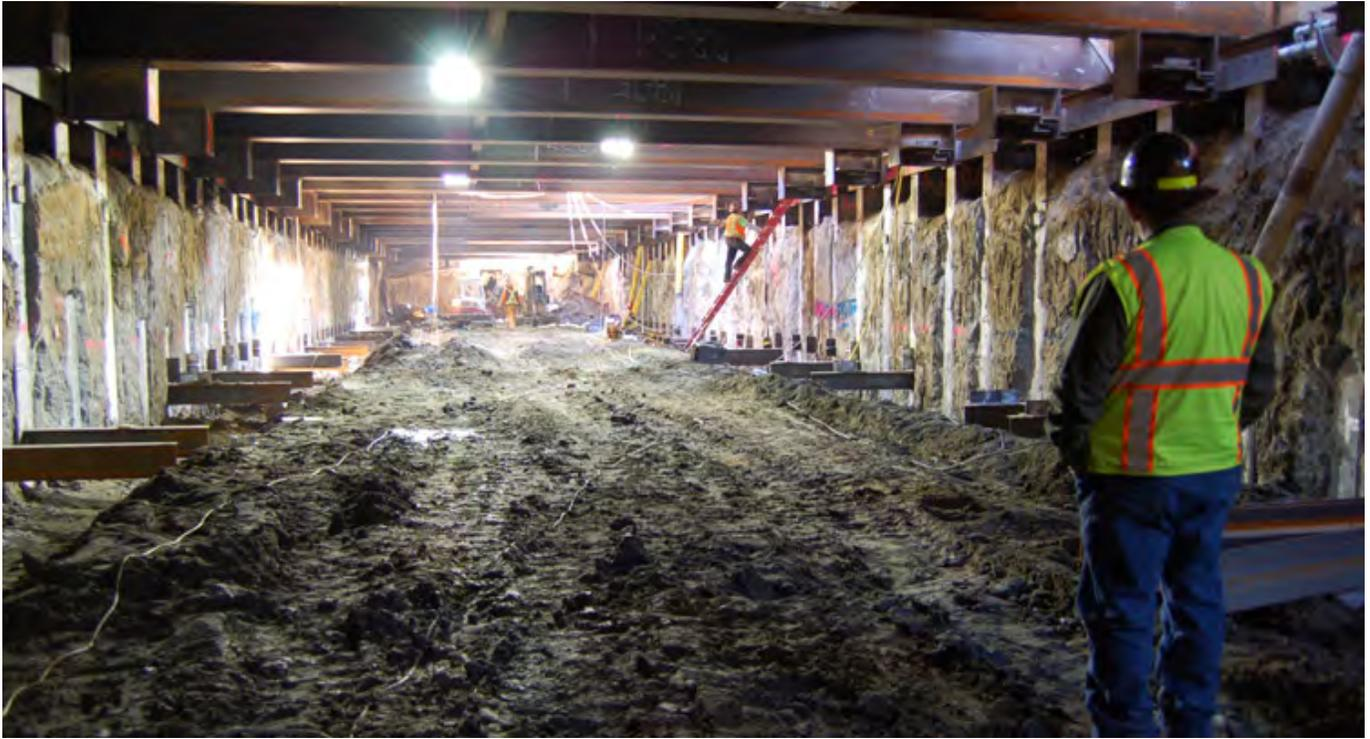
*A safety inspector surveys the launch box site at 4th Street in SoMa. Excavation work is ongoing and bracing is installed as material is removed.*
