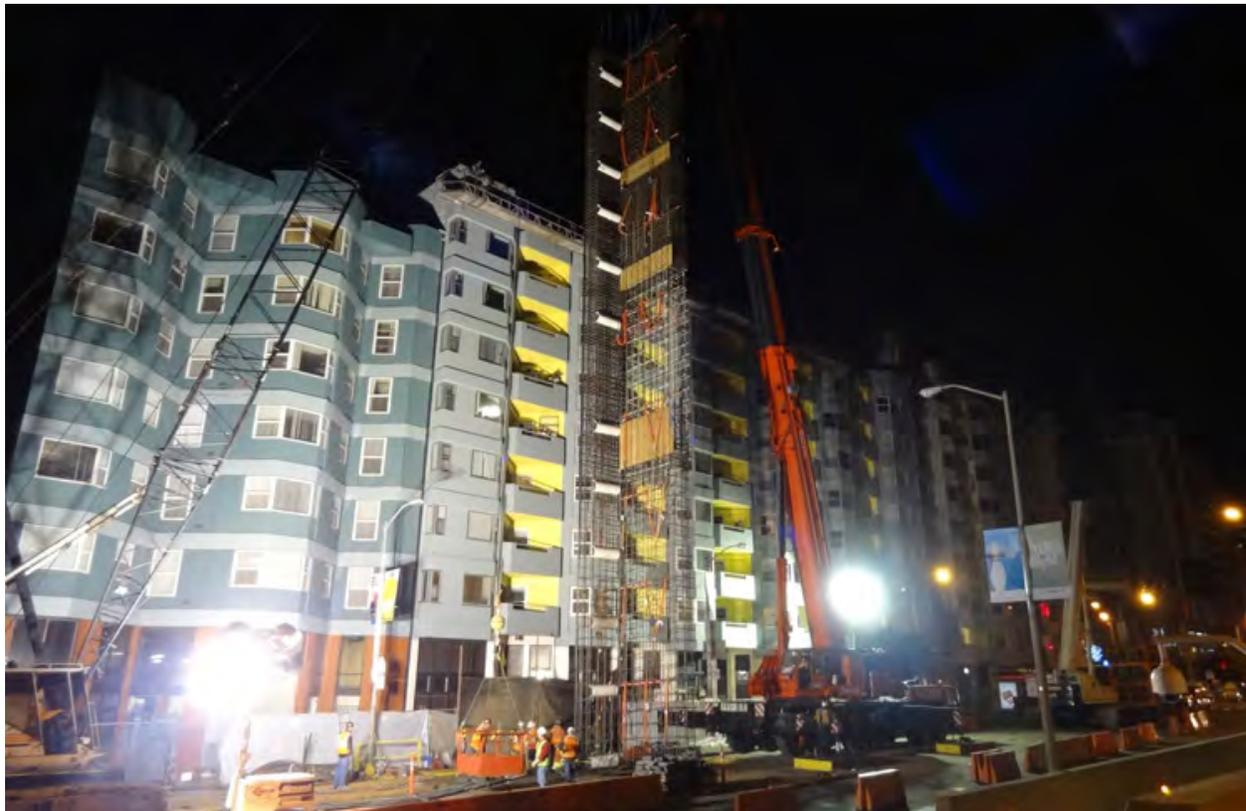
*Crews at the future Yerba Buena/Moscone station site lower one of many rebar cages into place prior to pouring concrete for the station headwalls.*
