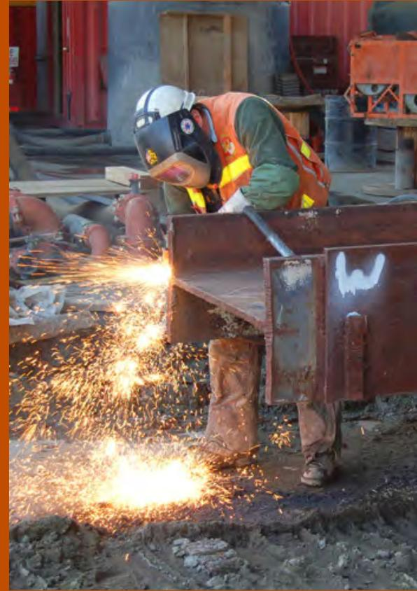
*A welder works on bracing that will be used to support the walls of the launch box on 4th St.*
