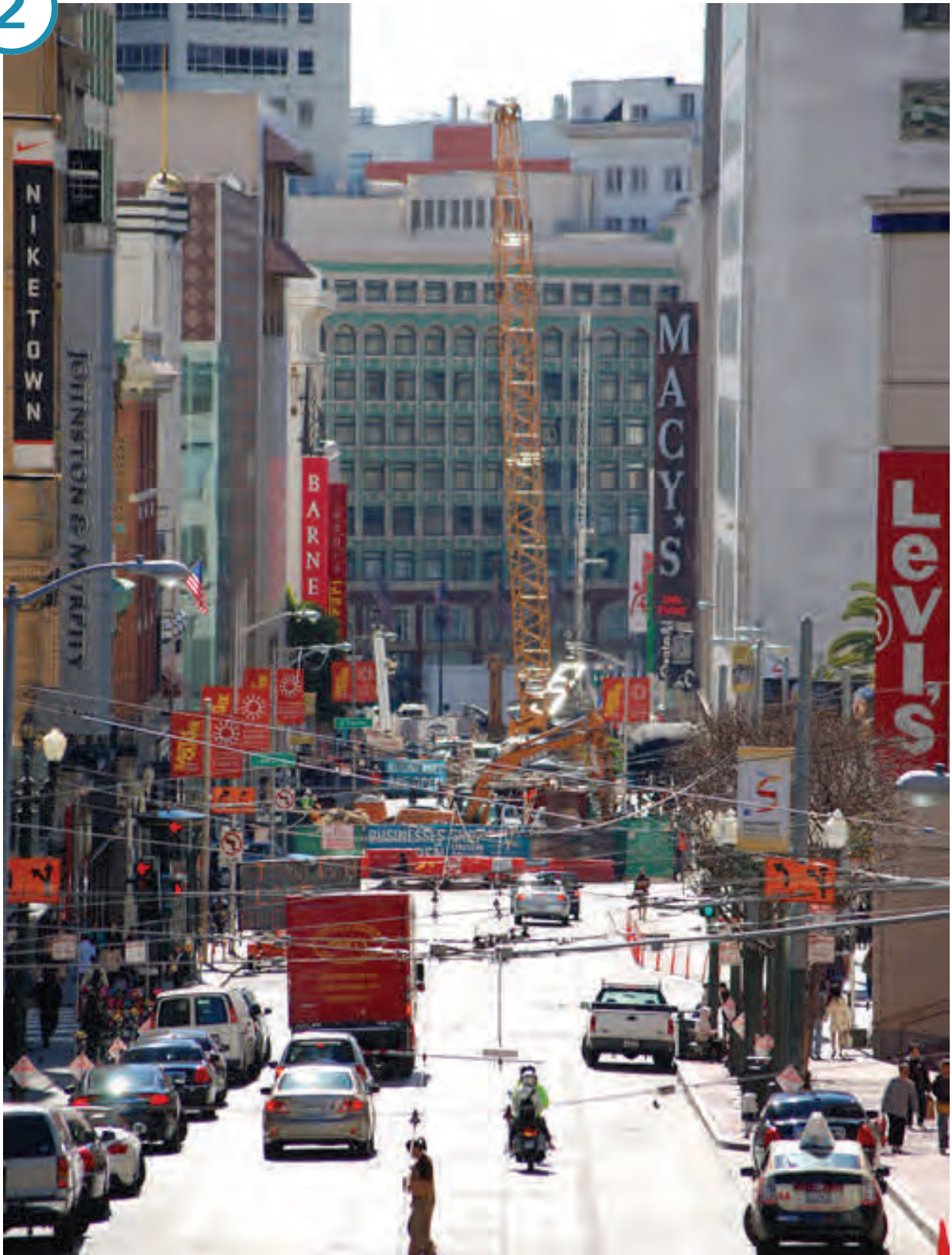
Looking south down Stockton Street from above the entrance to the Stockton Street Tunnel, toward the Union Square/Market Street construction site between Geary and Ellis, where station headwall construction is underway.
