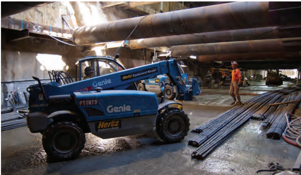
Crews have begun bringing in rebar that will be used to reinforce the floor slab of the launch box.
