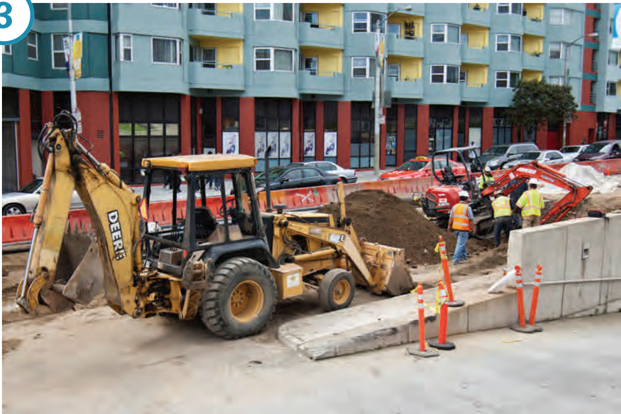
Headwall construction at the Yerba Buena/Moscone Station site has paused temporarily for workers to relocate a large-diameter water line.
