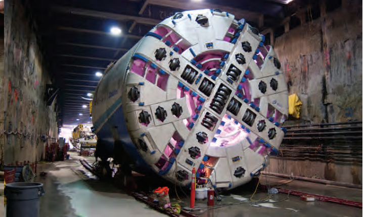
The first “ring” of the shield portion of tunnel boring machine Mom Chung arrived at the launch box work site in late April. Workers first had to bring the ring upright, before lowering it into the launch box onto a temporary steel cradle.
