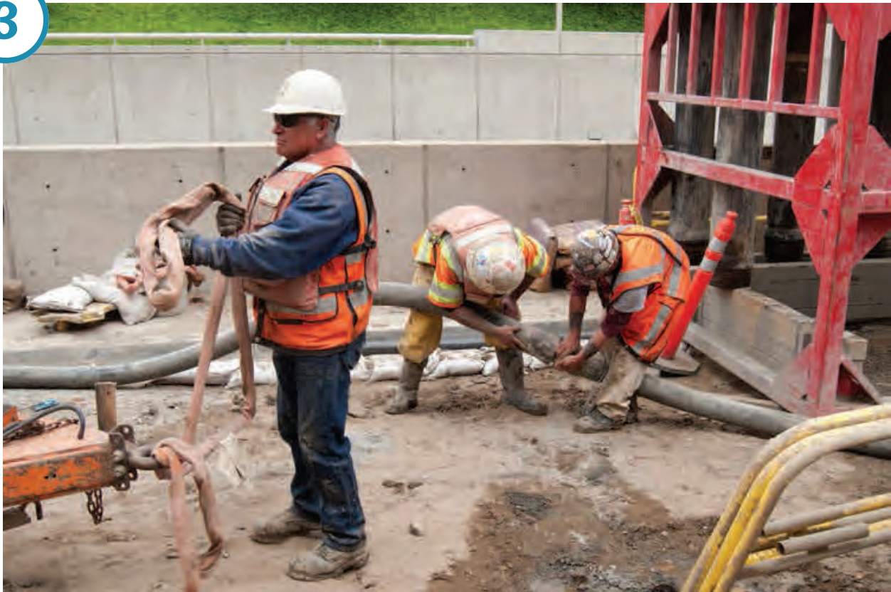
Headwall construction at the Yerba Buena/Moscone Station site.
