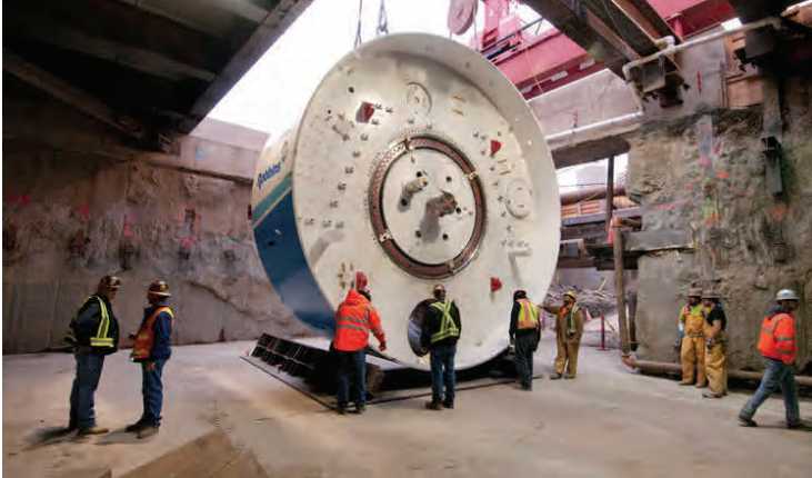
The first “ring” of the shield portion of tunnel boring machine Mom Chung arrived at the launch box work site in late April. Workers first had to bring the ring upright, before lowering it into the launch box onto a temporary steel cradle.
