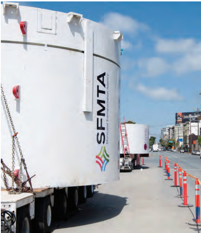
Segments of the forward “shield” portion of tunnel boring machine Mom Chung have arrived at the 4th Street launch box site. These “rings” are being lowered into the site one at a time, before being re-assembled.
