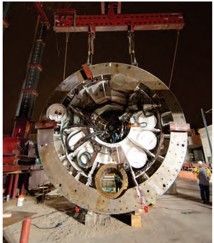
Segments of the forward “shield” portion of tunnel boring machine Mom Chung have arrived at the 4th Street launch box site. These “rings” are being lowered into the site one at a time, before being re-assembled.
