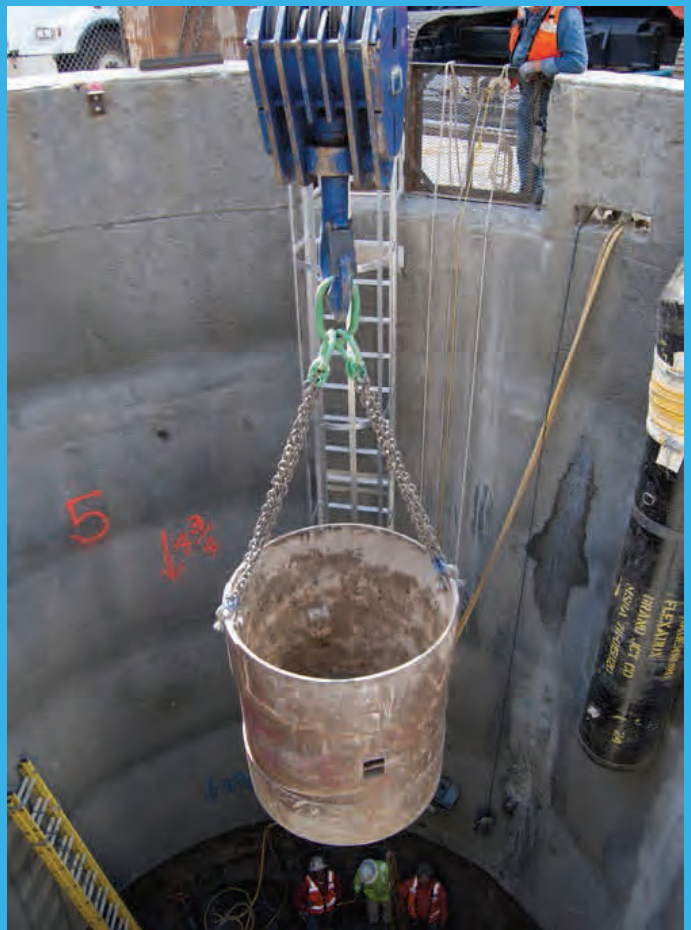
Above - Crews use a large steel bucket to remove spoils excavated from the large-diameter shaft currently being excavated at Ellis and Stockton.
