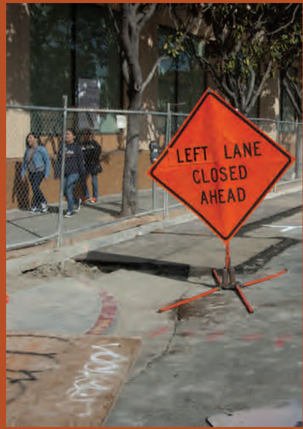
Work is near an interim completion stage on 4th Street between Folsom and Harrison, installing subsurface piping used in compensation grouting.
