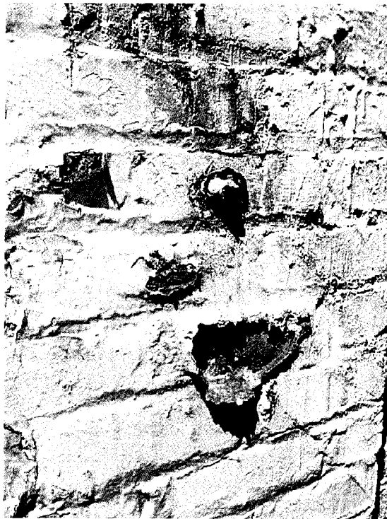
Figure 30. North façade, detail of spalling brick, April 2007. Source: Page & Turnbull, Inc.
