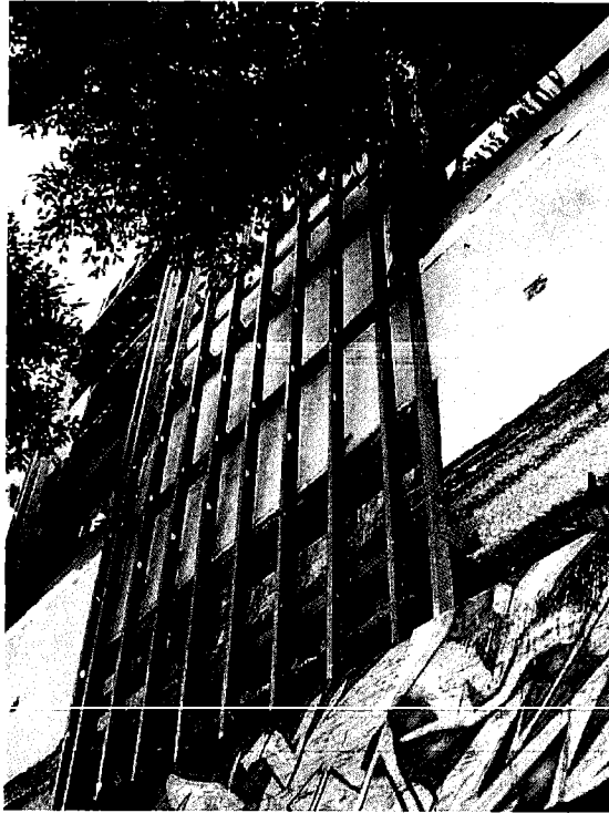
Figure 25. Primary (east) façade, detail of exposed steel and wood, April 2007. Source: Page & Turnbull, Inc.
