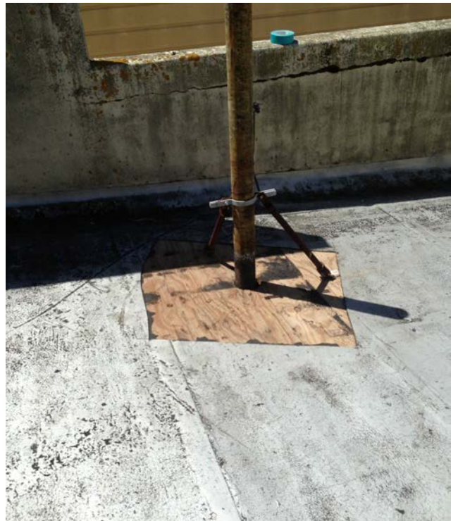
Penetration 2 – ACM Removed
