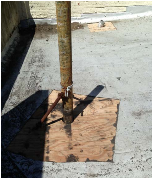
Penetration 1 – ACM Removed
