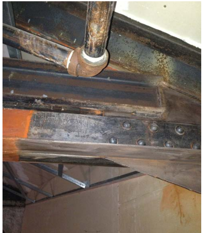
North side beam
