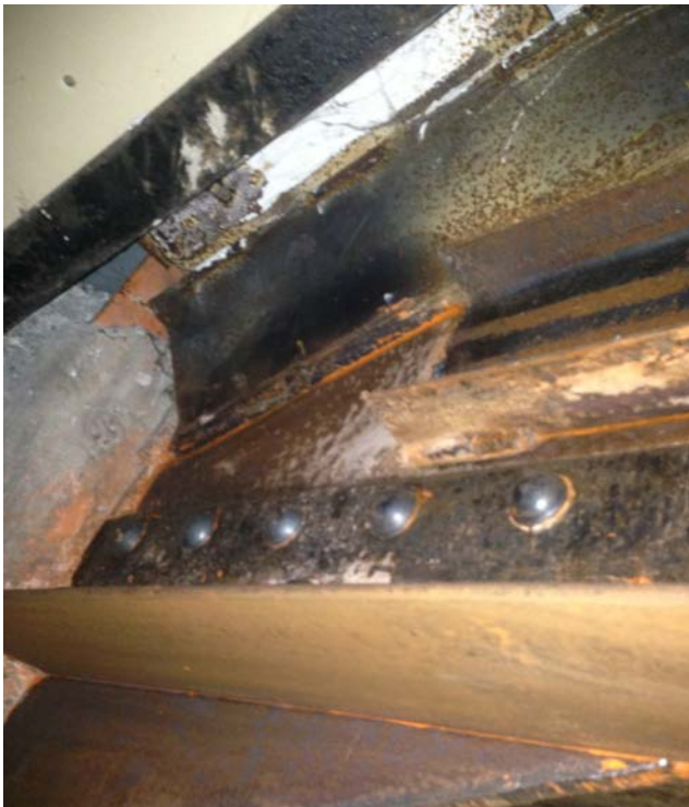
South side beam
