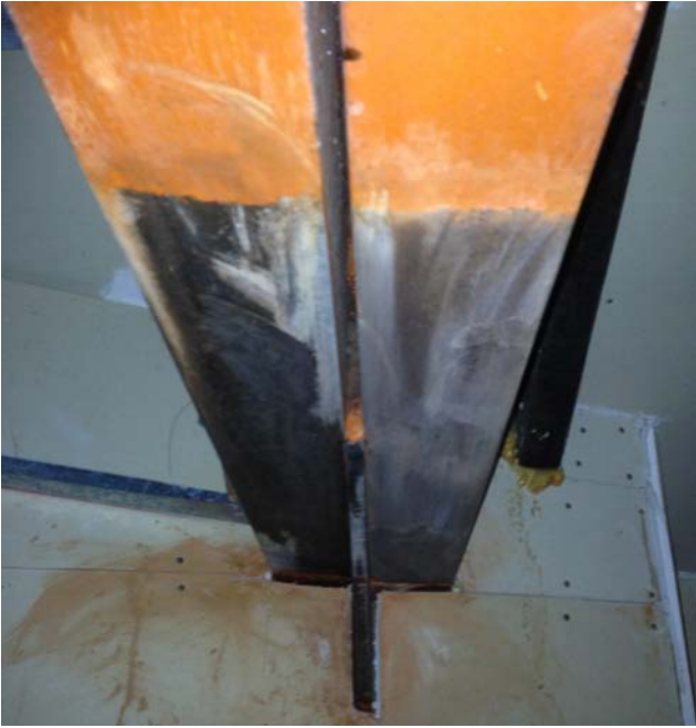
North side beam
