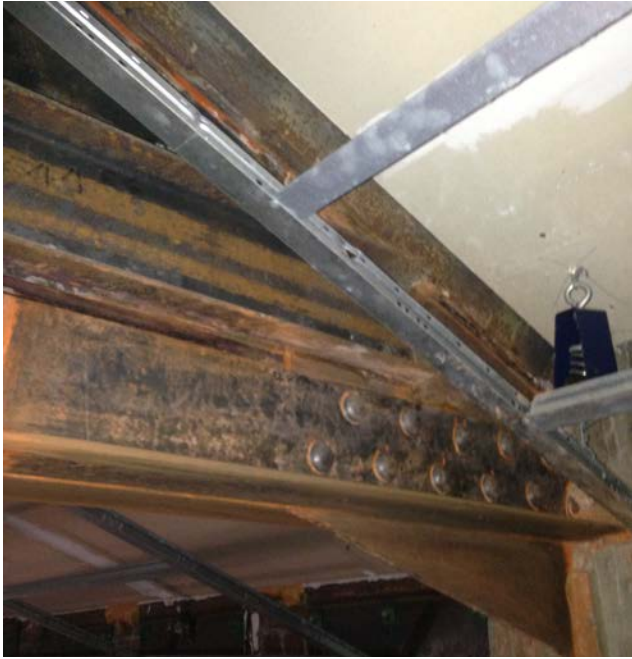
South side beam
