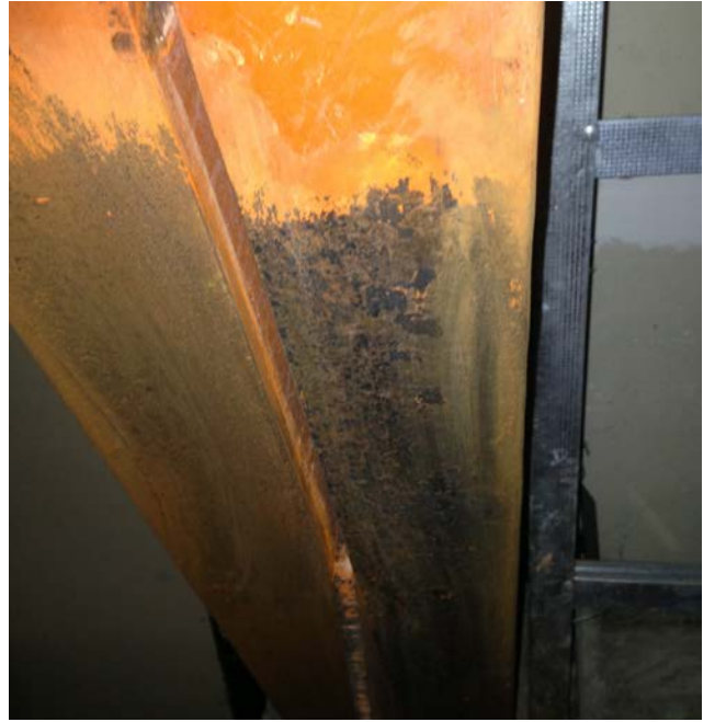
South side beam
