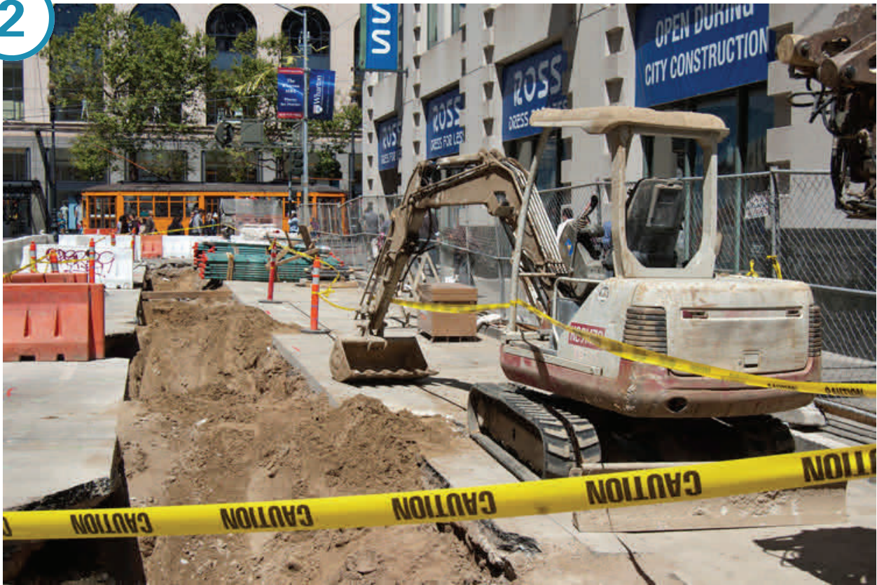
4th Street between Market and Stevenson, preparations for compensation grouting.
