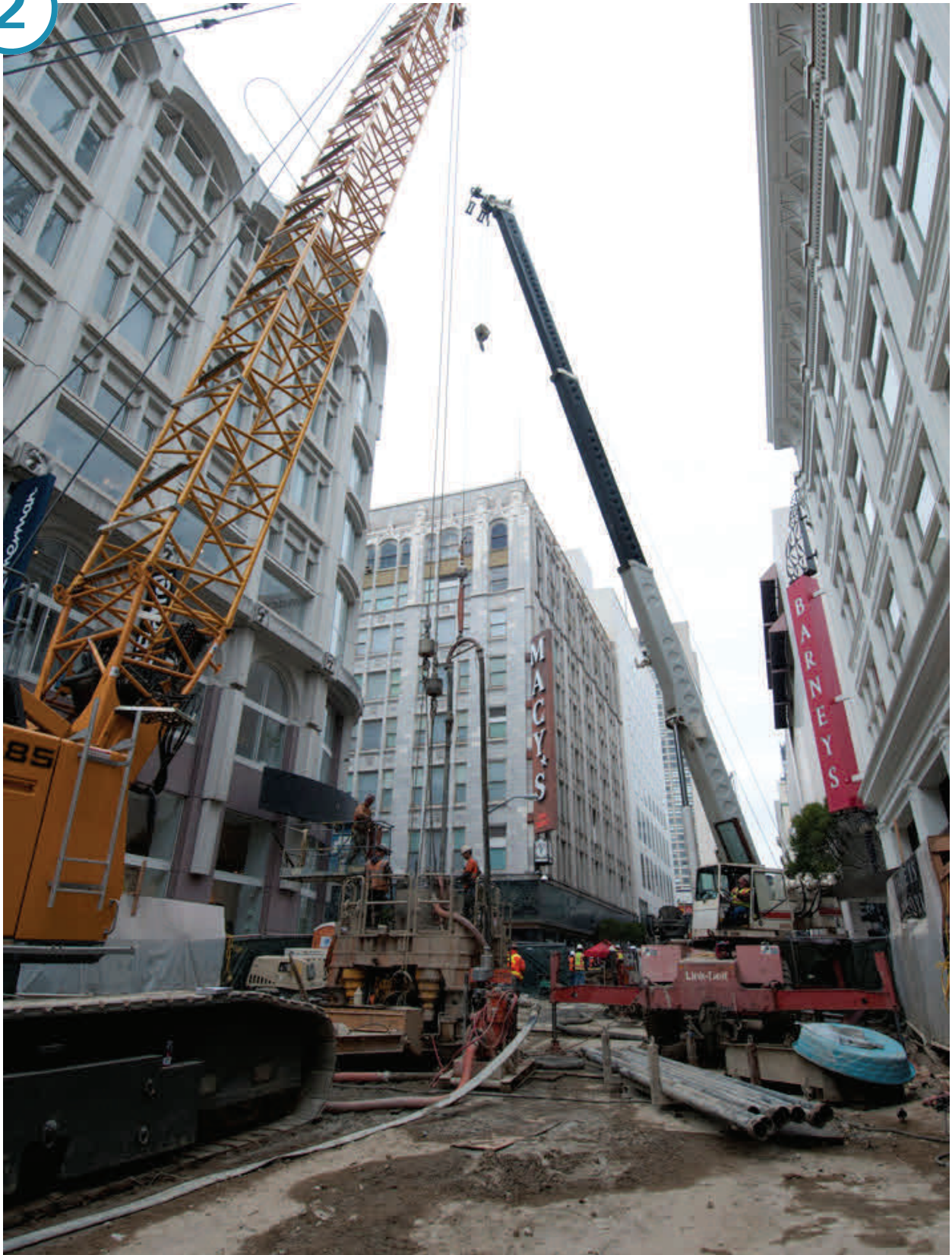
Looking north up Stockton Street, toward O'Farrell. Crews are excavating interlocking, subsurface shafts that will form the headwalls of the future Union Square/Market Street Station.
