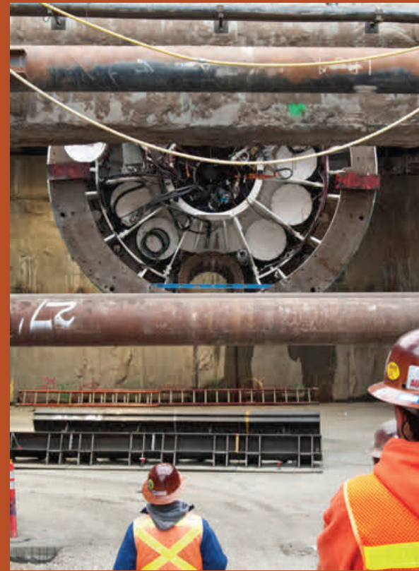
Workers monitor progress the TBM Mom Chung is lowered into place at the launch box ramp.
