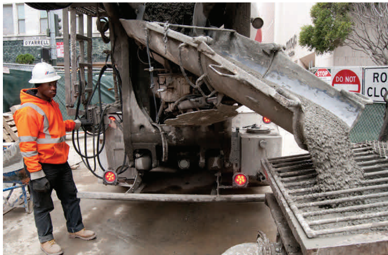
Concrete pour for Union Square/Market Street station headwall pile, south of O'Farrell.
