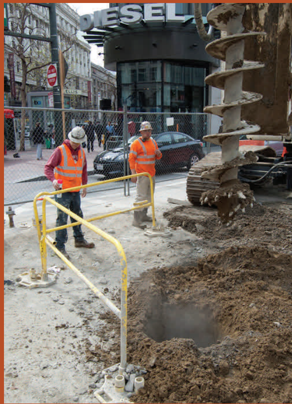
Workers performing drilling operations head of building the large vertical shaft at the corner of Ellis and Stockton.
