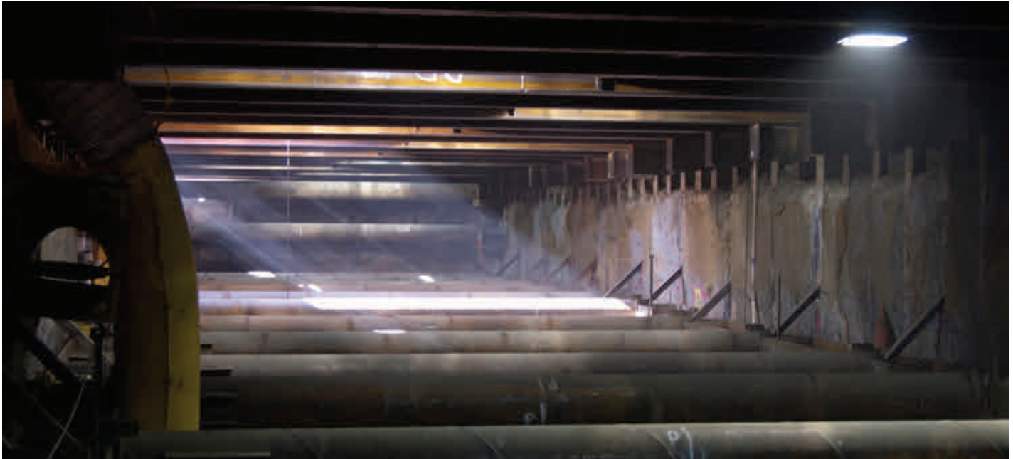
View looking north at the tunnel boring machine launch box site, showing temporary supports in place.
