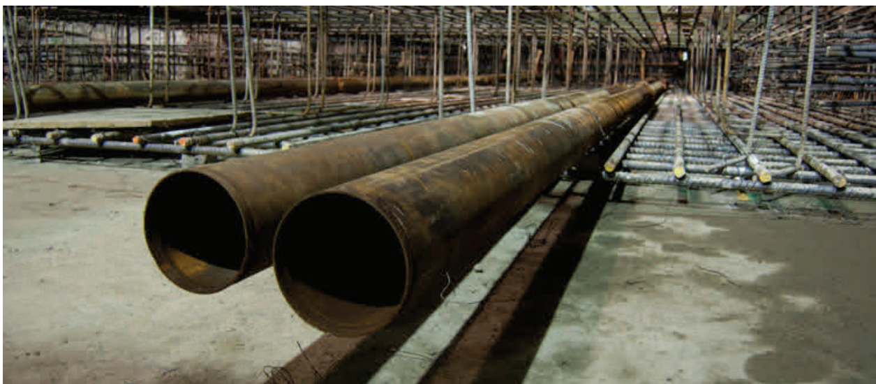
A close-up of piping and rebar that will reinforce the launch box floor slab.
