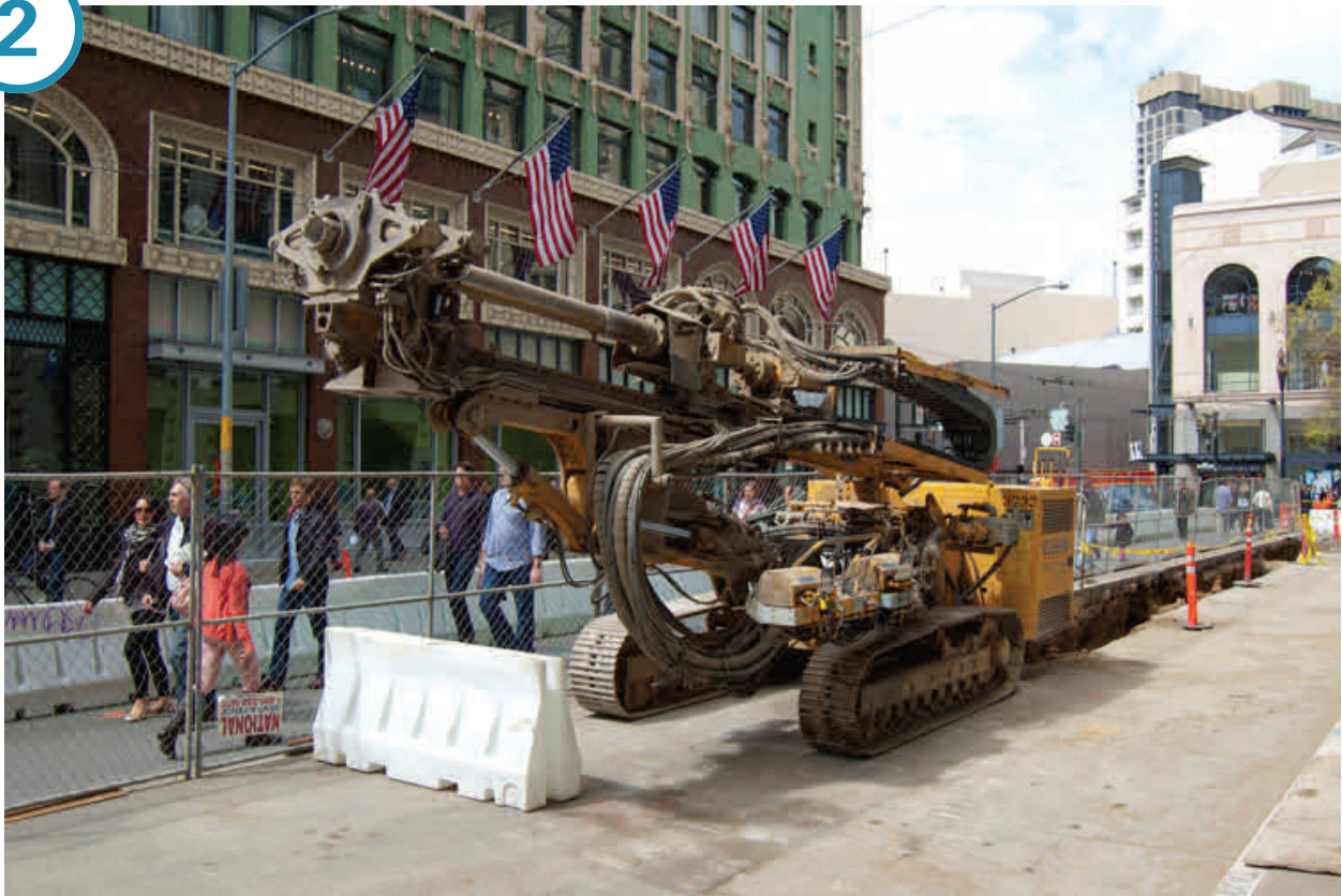
4th Street between Market and Stevenson, where preparation for compensation grouting will soon begin.
