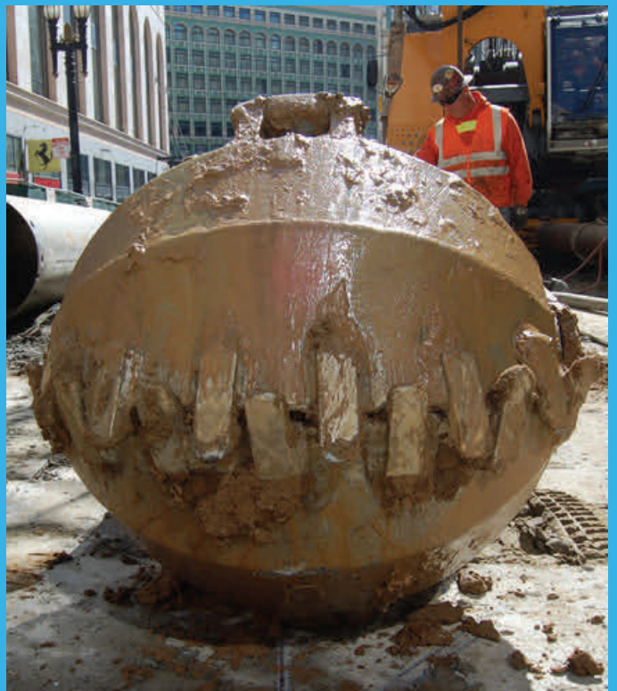
Below - A close-up of the clamshell bucket excavator used to dig the secant pile shafts used in the southern Union Square/Market Street Station headwalls.
