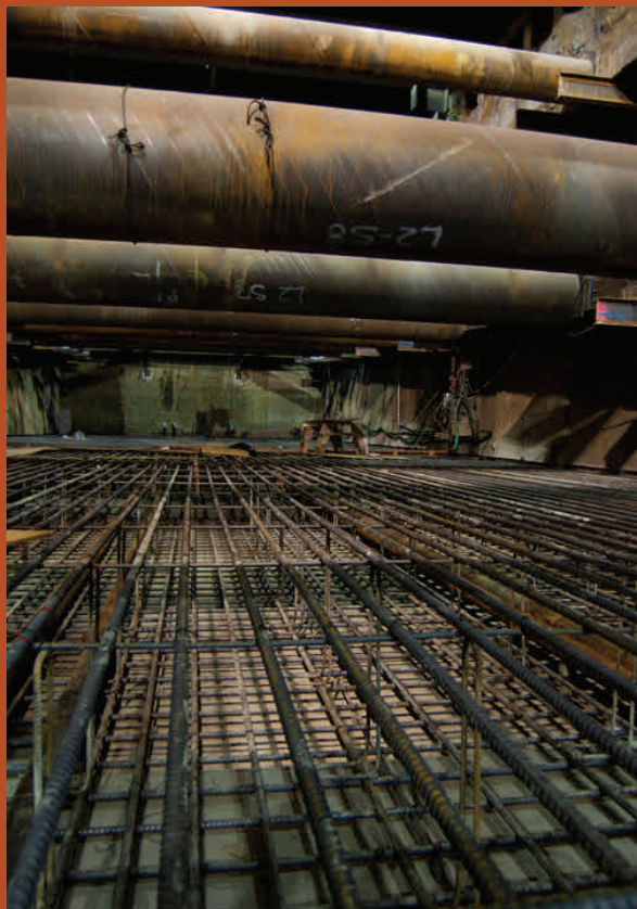
Looking north in the TBM launch box, with temporary supports above, and rebar for the future floor slab below.
