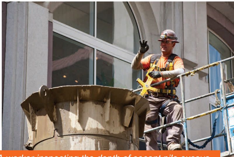
A worker inspecting the depth of secant pile excavation for the Union Square/Market Street headwalls.
