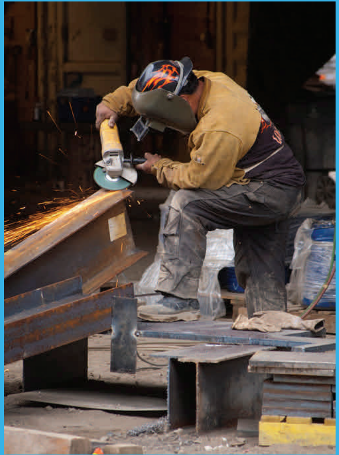
Above - A worker uses a grinder while fabricating temporary supports that will be used to shore up the launch box before the floor slab is poured.
