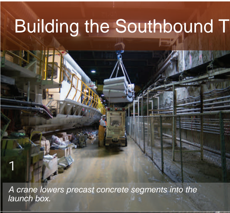
They are transported to the tunnel boring machines by using a tunnel service vehicle (TSV)
