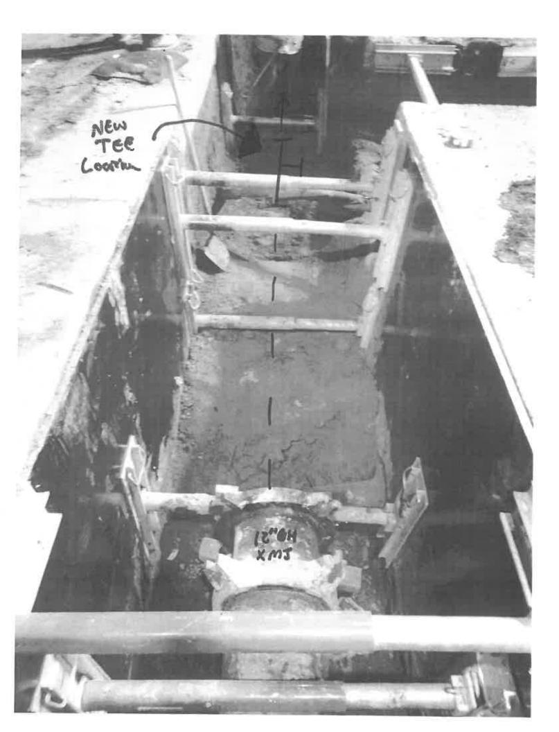
Remove remainder of existing pipe in added area, excavate remainder of hydrant lateral, install added piping, install hydrant offset, backfill added mainline section & lateral, concrete and asphalt pave added mainline section and lateral, re-backfill old mainline section, continue shoring rental for added trench, sawcut, excavate and support 3" steel line.
