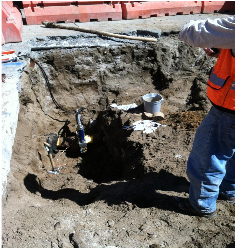
Repairs being made to the damaged gas line.
