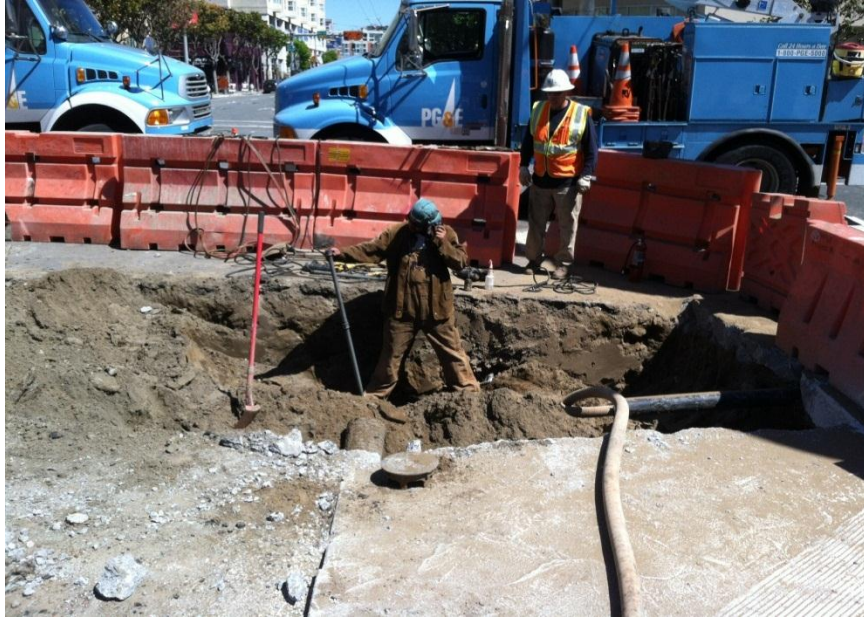
PG&E performing repairs on Sunday after the gas was turned off.
